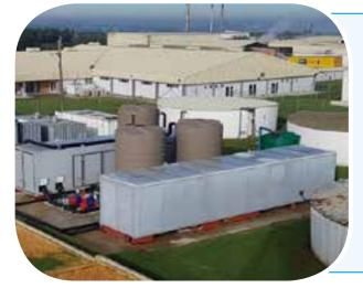
In F2017, County Fair partnered with a supplier and designed a 2.8 million litre per day tertiary water treatment plant for the second largest poultry processing facility at County Fair Hocroft. The water treatment plant utilises aqua mobile ultrafiltration and reverse osmosis technologies to provide County Fair with potable water for re-use in production. The reverse osmosis water treatment plant was commissioned in October 2017.
